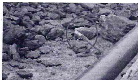
Fixed type DS system at Coal Yard
