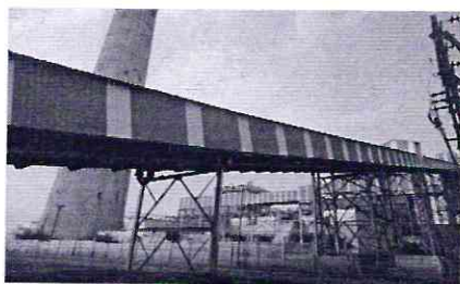
Closed type coal conveying system
